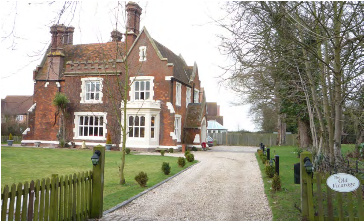
Picture 1.27 The Old Vicarage seen from the Street
