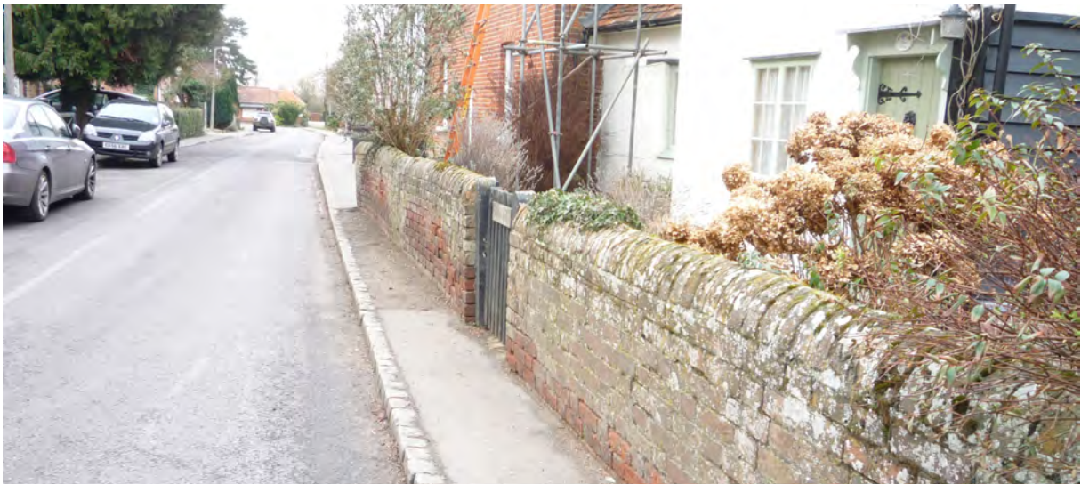
Picture 1.5 Red brick front boundary wall to Tye Cottage and granite kerbing, The Street
