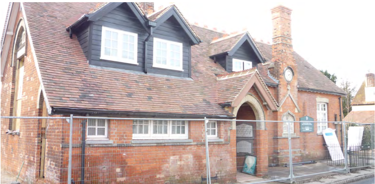
Picture 1.12 Former Memorial School, with works ongoing
